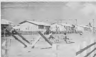
The swing swing, the inter-lectors' lecture, and the merry-go-round which in the playground recently installed by the Home Building Foundation at the new housing development north of the Lago Sport Park. Set away from street and completely fenced, it offers an ideal play-place for the small boy. A duplicate set of equipment is scheduled to be installed at Eusebio, the center group at Home Building Foundation houses.
